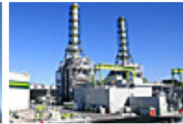
Kawasaki Natural Gas Power Generation Co., Ltd.
