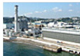
Tokyo Gas Yokosuka Power Co., Ltd.
