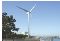
Wind power facility at Sodegaura LNG Terminal
