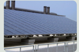
Solar panels installed at Keihanna Technology Innovation Center produce 48,000 kWh of power per year
