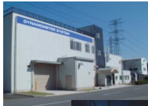
Dynamometer Systems Research and Development Building
