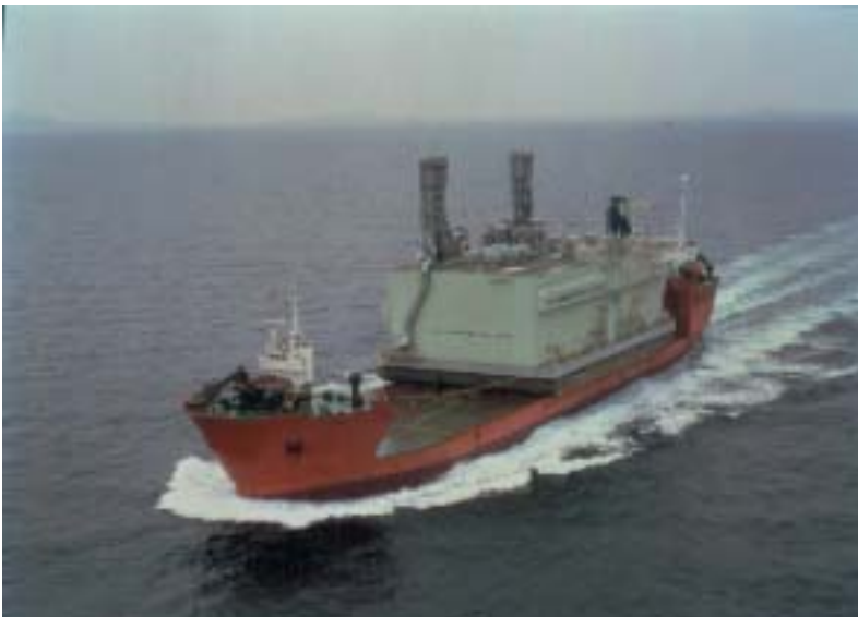
19MVA low-speed diesel-engine generator facility
