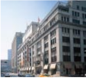
Nihonbashi Main Store (Main Building)
