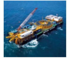
Laying a submarine transmission cable
