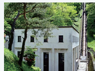
Uwanoshiro Power Plant
