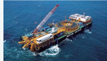
Construction of submarine power transmission lines
