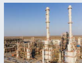
Gas to Gasoline Plant (トルクメニスタン)
