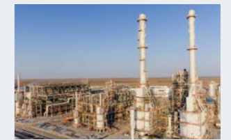
Gas to Gasoline Plant (トルクメニスタン)
