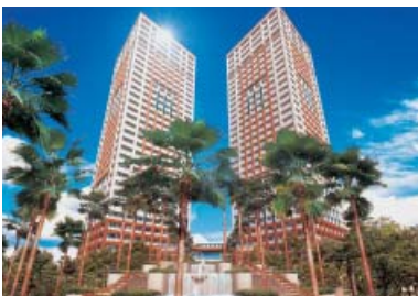
External view of AIR RESIDENCE Shin-Urayasu Premium Towers
