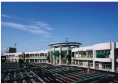
External view of Mallage Kashiwa
