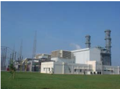
Phumy III power plant in Vietnam
