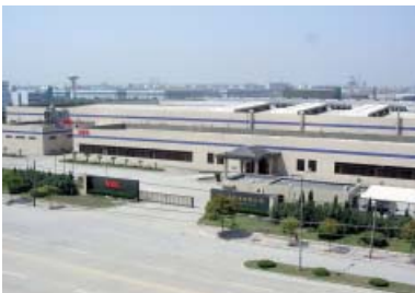
The Kunshan plant, a joint-venture operation with NSK Co., Ltd., and NSK's flagship production base in China.
