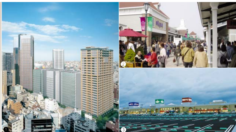
① Tokyo Residence—High-rise condominium located within “I-Garden Air,” an urban development in Tokyo ② Sano Premium Outlet—Nissho Iwai’s third premium outlet, based on the image of the U.S. East Coast and featuring approximately 80 shops ③ Mallage Saga—Suburban commercial facility development, featuring parking for 3,000 vehicles
