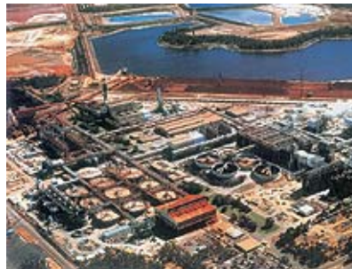
At the Worsley Alumina Project in Australia, of which Nissho Iwai has a 7.5% share, production capacity of alumina has expanded to 3.1 million tons per year.
