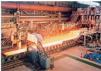
A hot-rolling plant The company enables efficient connections between plants and steel products users.
