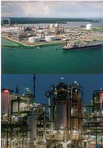
A plant owned by P.T. Kaltim Methanol Industri, an Indonesian methanol manufacturer in which the Company has a stake
