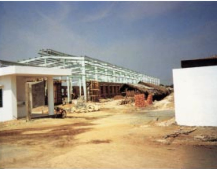
The Vietnam Japan Aluminium Co., Ltd. (VIJALCO) factory under construction.
