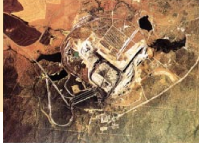
Coal pulverization and loading facilities
