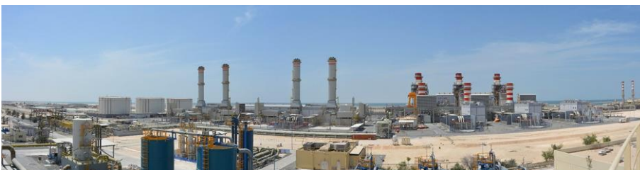
[Mirfa power and desalination plant]
