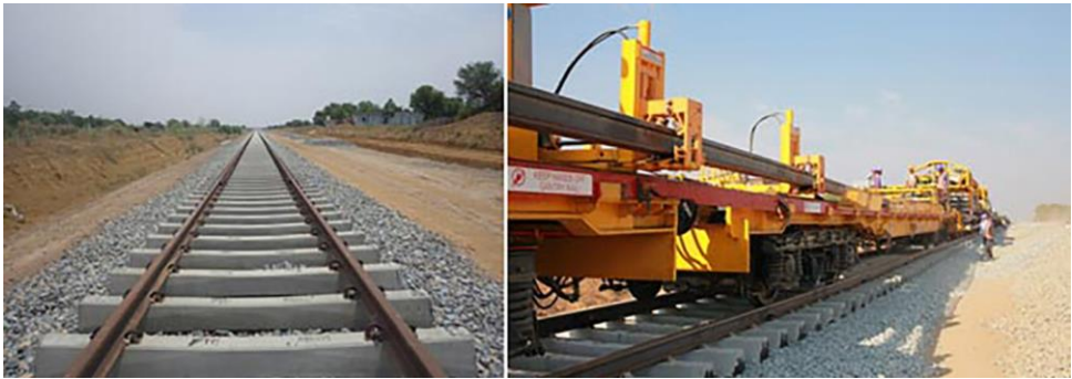
At the track laying site
