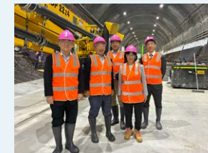
Independent directors touring site of expressway construction project in Australia for which an order was received by Capella Capital Pty Ltd
