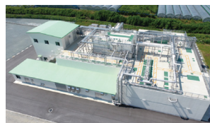
New wastewater treatment plant at the Kyushu Factory
