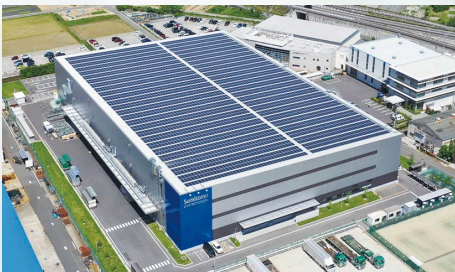
DT-SBU Factory2, Nagoya Works
