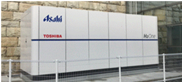
H 2 One™, a Self-contained System for Supplying Hydrogen Energy
