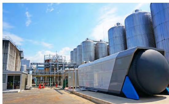
System to Generate Power from Biomethane-Gas-powered Fuel Cells
