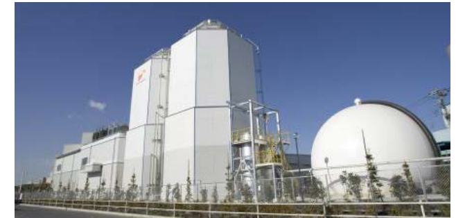
External View of Bio Energy Jonanjima Plant
