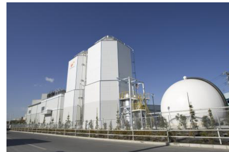
Methane fermentation system (Jyonanjima food recycling facility)
