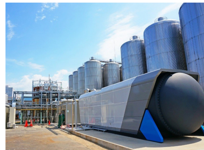
Biomethane gas-powered fuel cell power generation system
